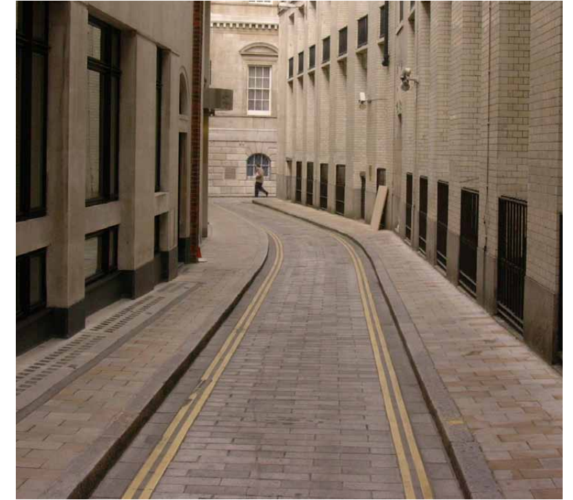
Retained raised kerb to carriageway
