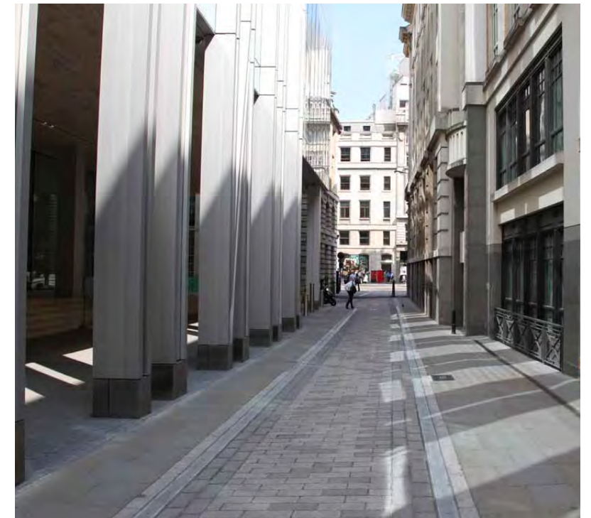
Raised carriageway with flush kerbline
