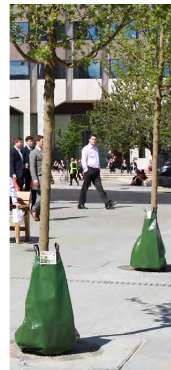
Treegators, as manual tree pit watering provision during establishment
