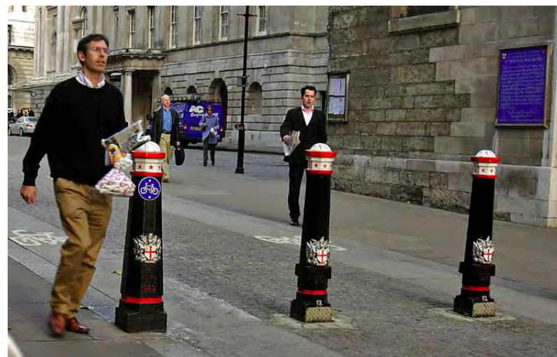
Bollard line with C3 demountable bollards
